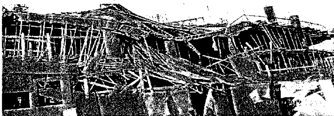
Collapsed Form work (New Library Building Project)
